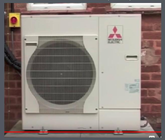
This machine uses energy in the "outside" air drawn across a coil again with a refrigerant and compressor to amplify the energy to produce hot water. Like a ground source heat pump this output is easily measured using a btu meter which makes thermal rec (TREC) recording possible.
