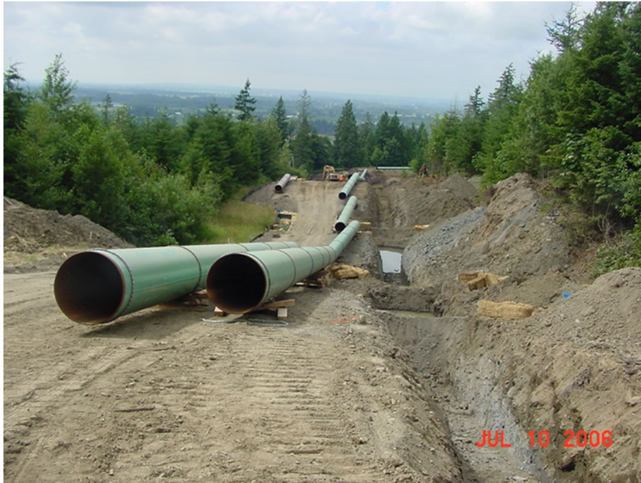
Figure 1 Transmission pipeline construction in the Northwest
