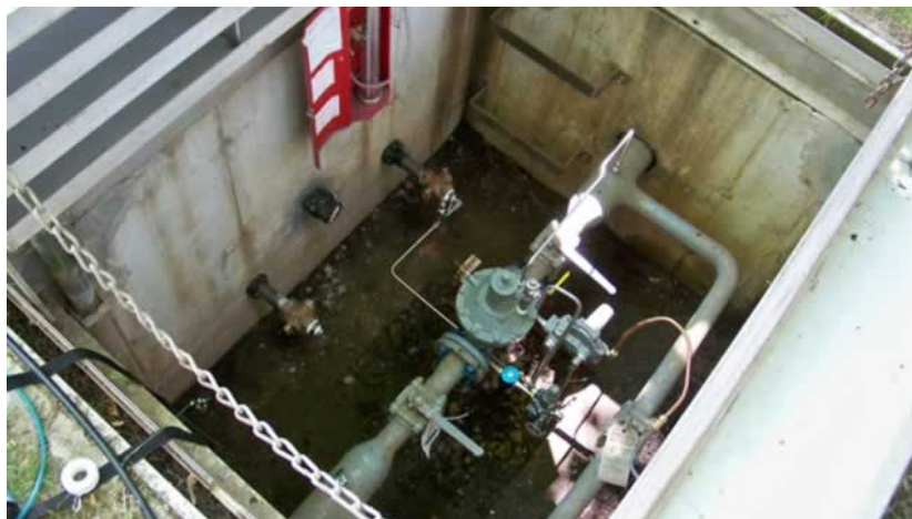
Figure 4 District Regulating Station –Vault Type
