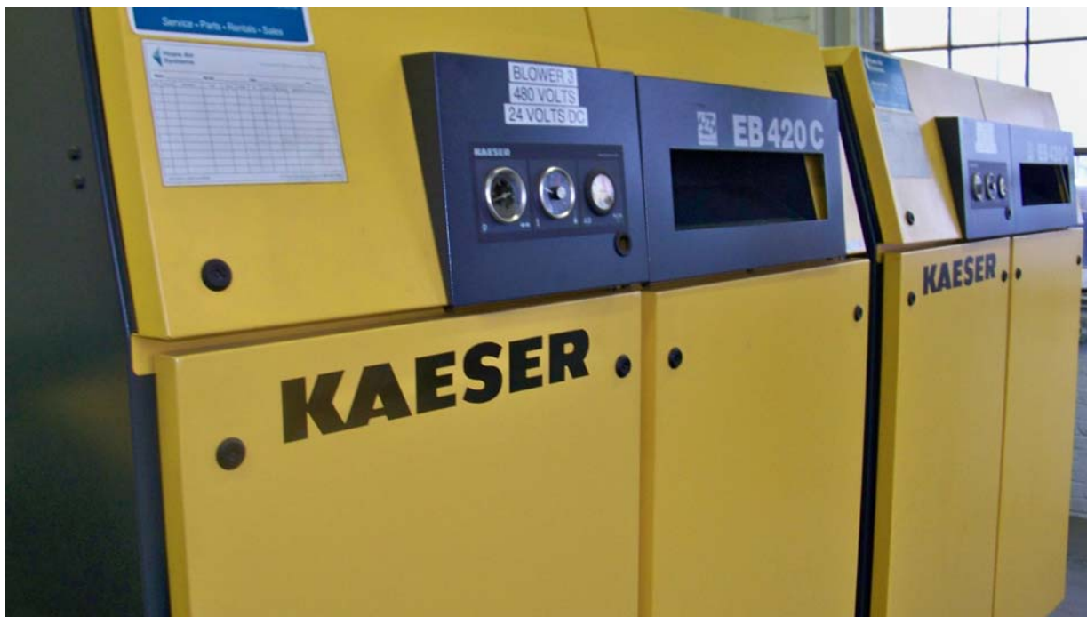
Liberty Keene – The plant mixes propane with air supplied by the blowers shown above.
