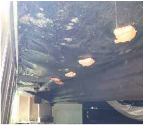
SPF belly patch: Installers use SPF to patch access holes in a mobile-home belly after blowing insulation.
