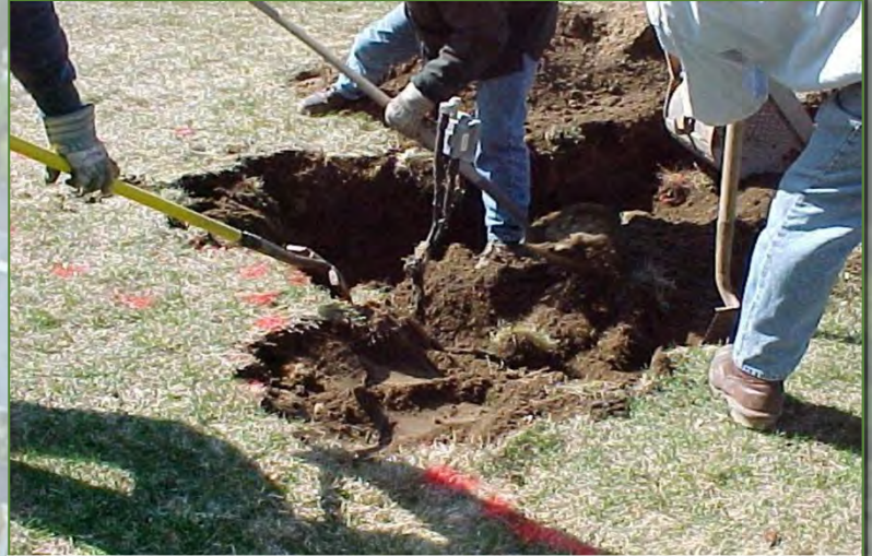
Practice Reasonable Care: Exposing Underground Facilities by first using Hand Tools before Digging with a Machine.
