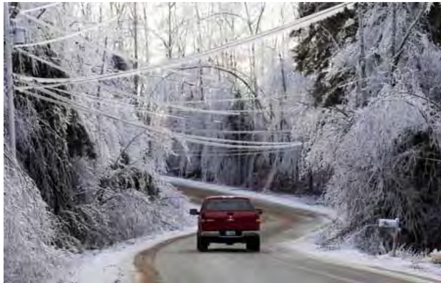
Figure V-2 - Ice loading on lines during December 2008 ice storm. (Photo courtesy of PSNH, location unknown.)
