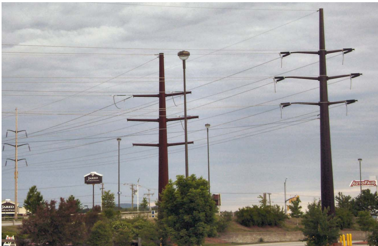
Figure IV-1 - 115kV transmission line structures located near Mall of New Hampshire in Manchester. (Photo by NEI – PSNH System)
