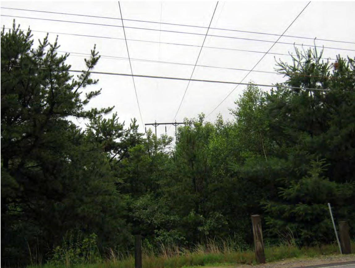
Figure V-12 - South view of circuit P145. (Photo by NEI)
