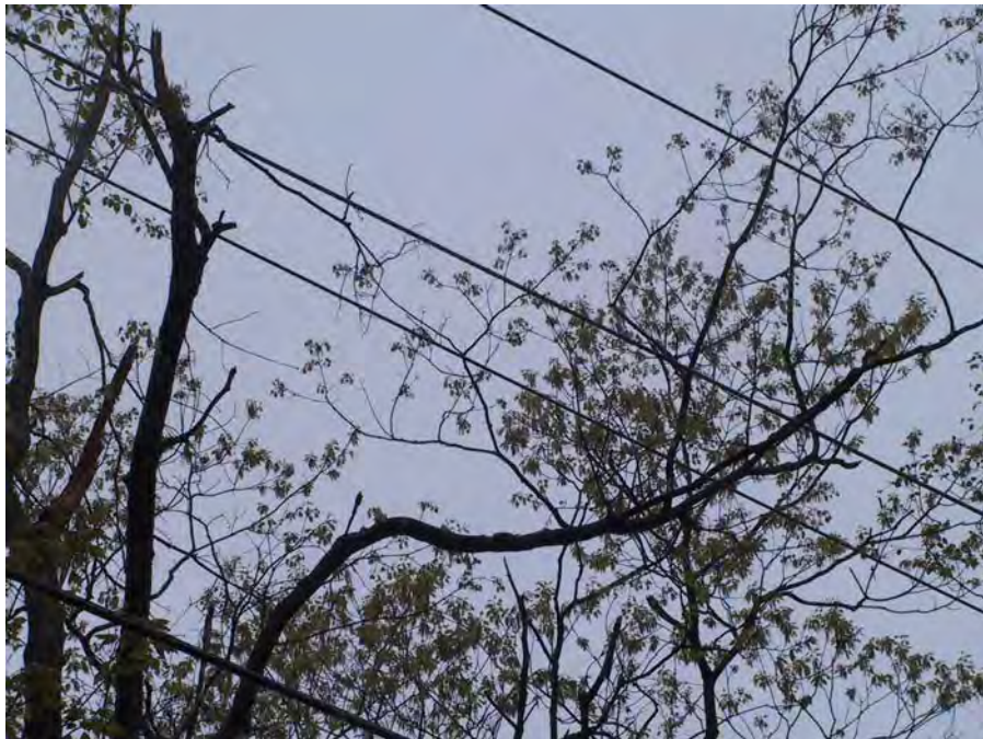
Figure V-5 - Small diameter immature trees broken above conductors in New Ipswich, NH. (Photo by NEI)
