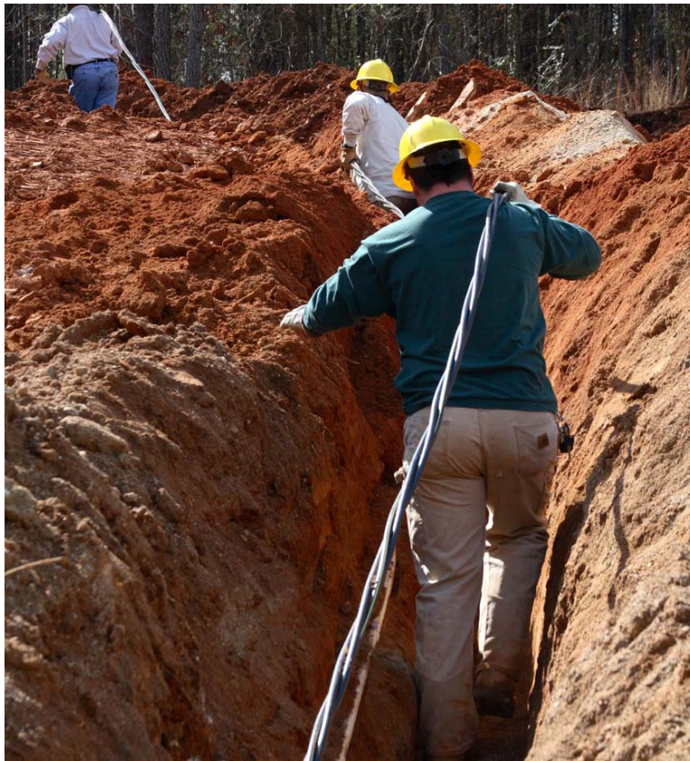
Figure B-2-Installing direct buried cable. (Photo courtesy of Southwire)
