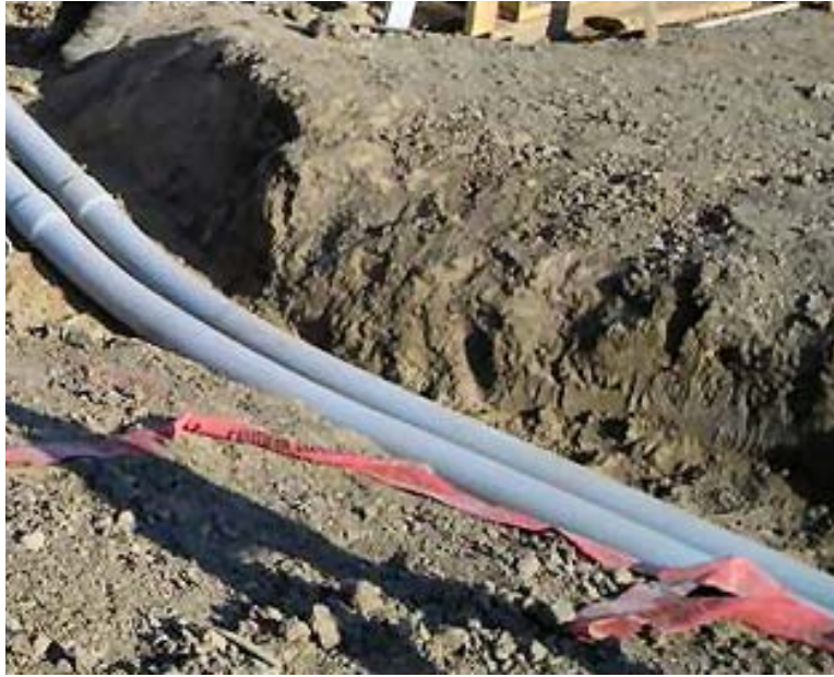
Figure B-5 - Conduit and Trench for Underground Distribution (Photo by NEI-Grand Prairie, Alberta)
