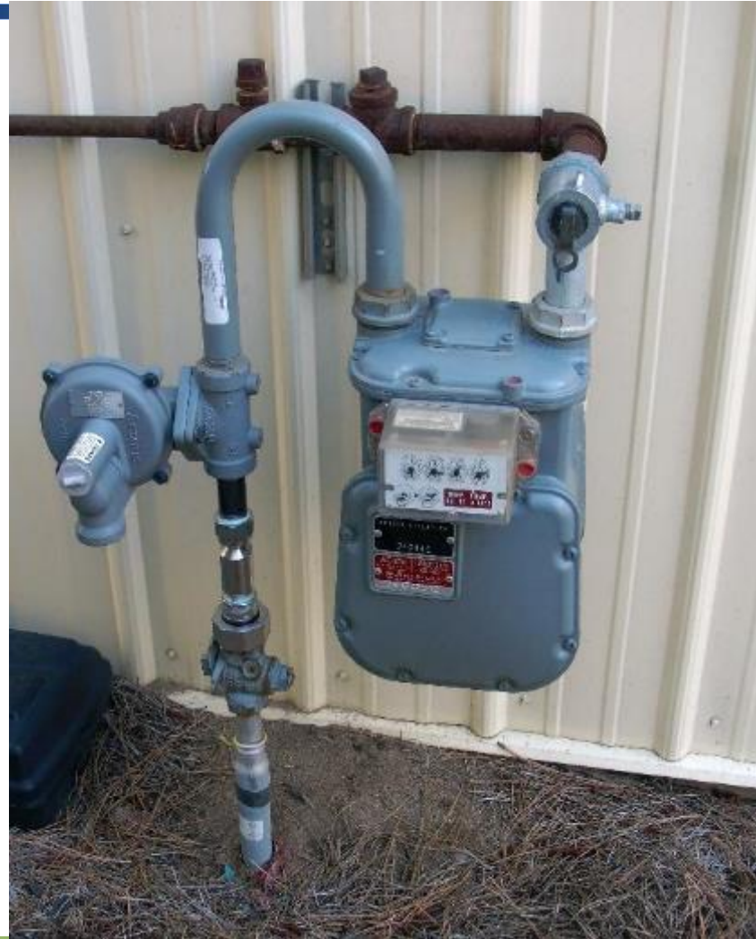
Meter set after breakaway installed 20
